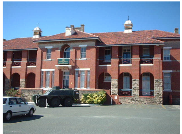
Heritage will be preserved in the Museum's expansion at Artillery Barracks
