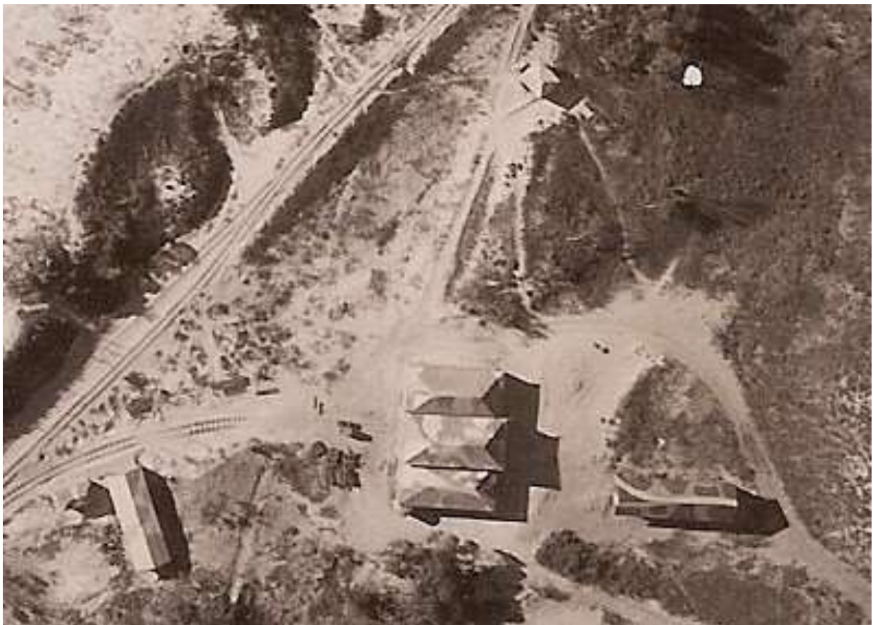
POL Store, Skedding Store, Workshop and Latrines at Oliver Hill
