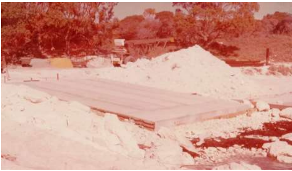
Fixed portion of the barge hard standing.
