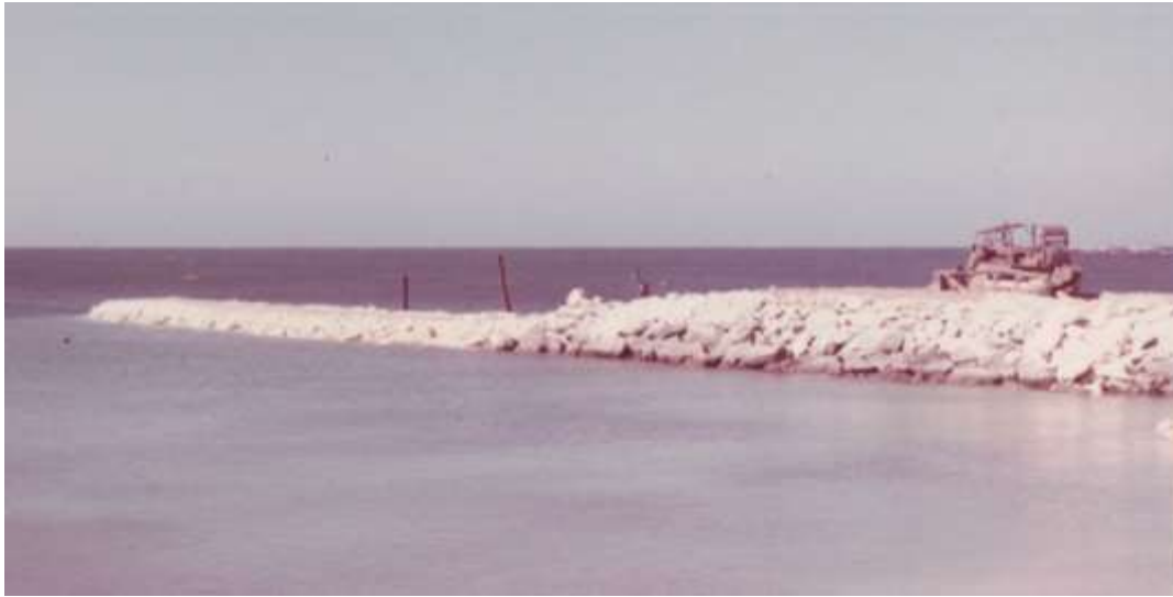
Levelling and compacting the groyne
