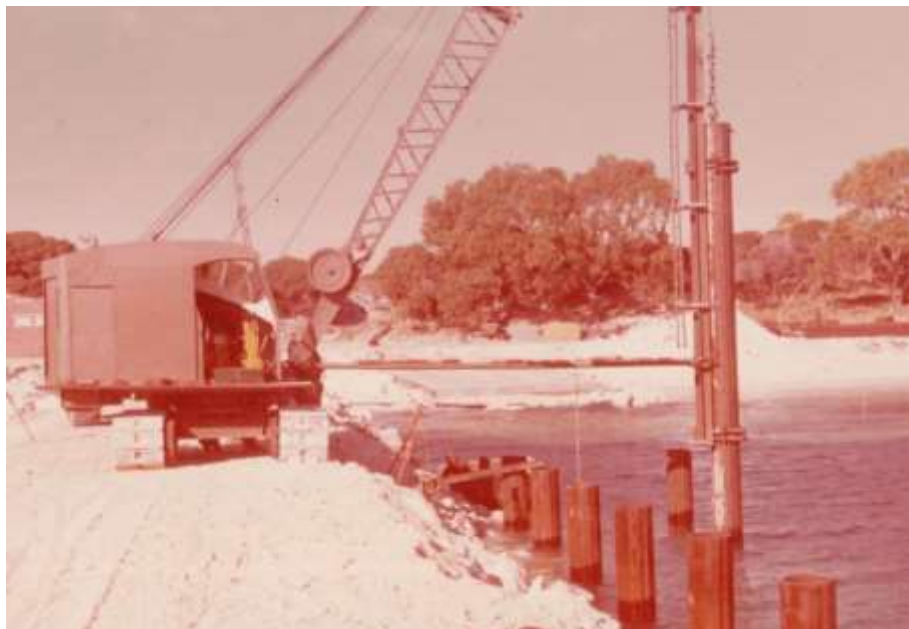
RB 23 driving piles
