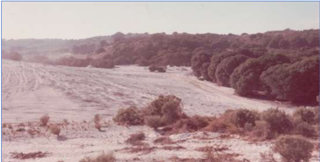
Reclamation works in progress.
