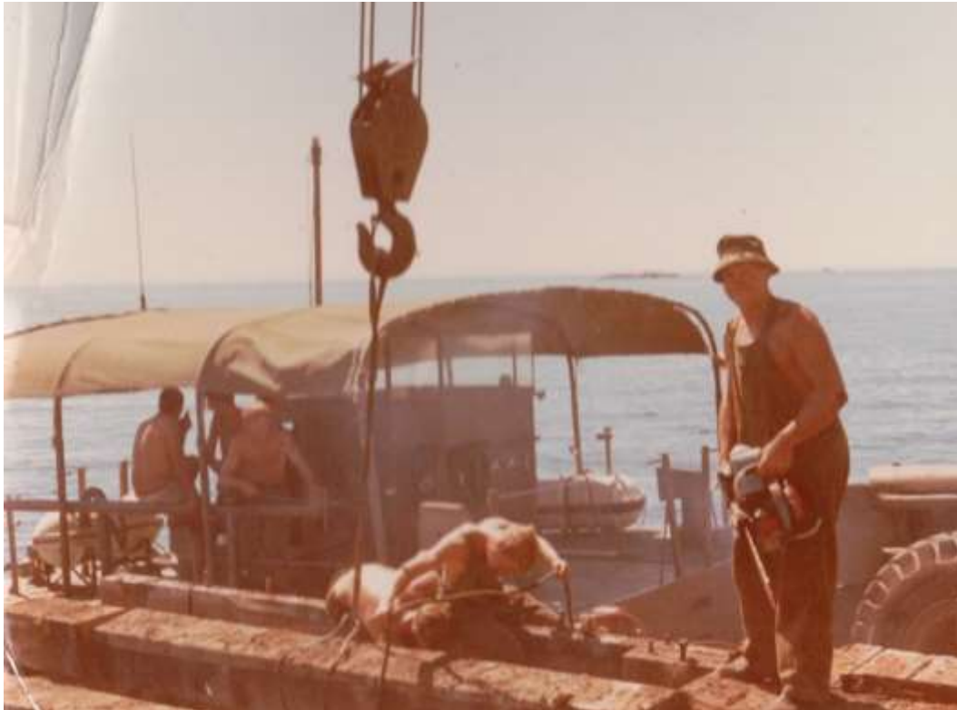
Army Jetty (1935, 1942) Rottnest in process of demolition 1972
