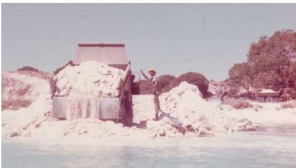
Dumping Class 2 stone to extend the groyne
