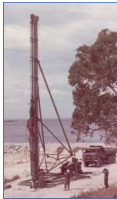
(L) Blasting operations (R) Pile driving frame assembled
